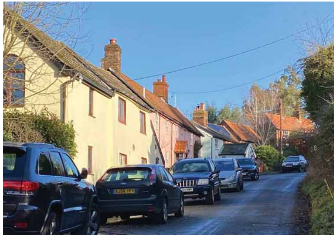
View looking up White Horse Hill with distinctive stepped arrangement of cottages.
