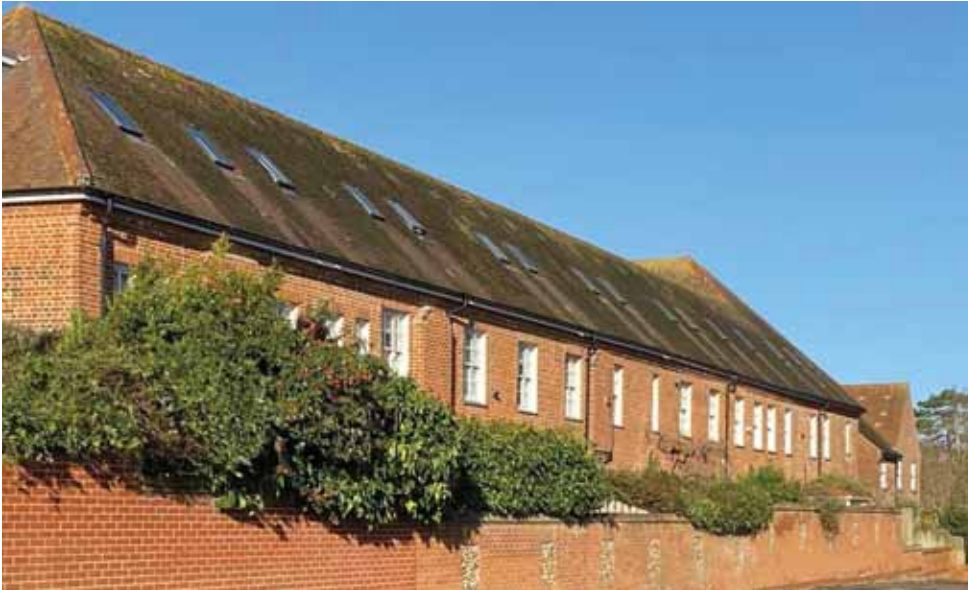
View north along Lemons Hill which is flanked by the brick wall and imposing building of the former Workhouse
