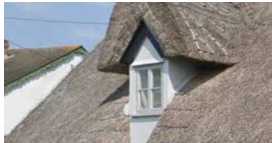
Timber framed roof windows
