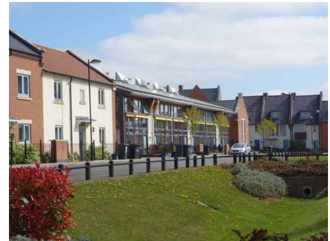
Figure 26: An example of a SuDS corridor - Upton Urban Extension, Northampton.
