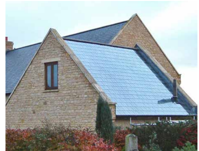
Figure 53: Positive example of integrating solar panels at the design stage.
