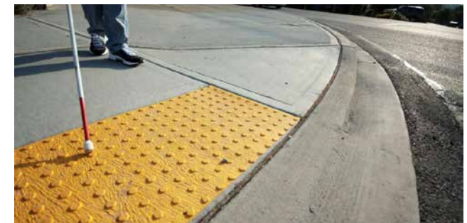
Figure 48: Example of tactile paving to facilitate movement for people with visual impairment.
